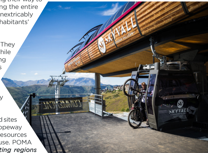
SKYVALL Valley Lift - Loudenvielle - FRANCE - 2019
